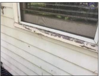
Plate 28 – Peeling paint around window frames at 60 Edmondson Avenue.
